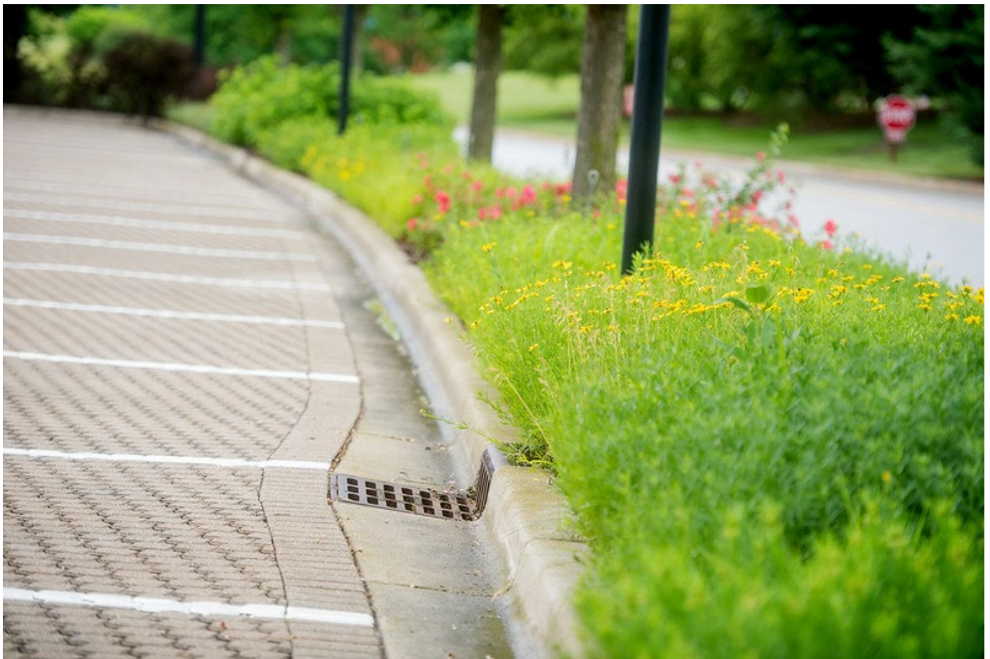
The Morton Arboretum's permeable paver parking lot and bioswales reduce flood risk and improve the quality of water in Meadow Lake. Photo credit: CMAP.
