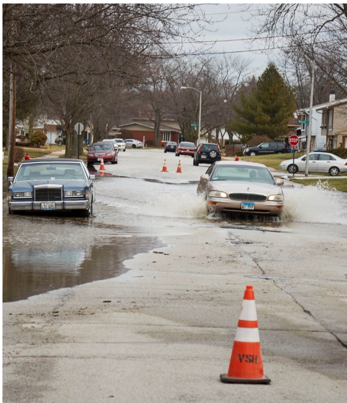
Many municipalities have developed stormwater management and resilience plans to reduce the impacts of urban flooding. Photo credit: CMAP.
